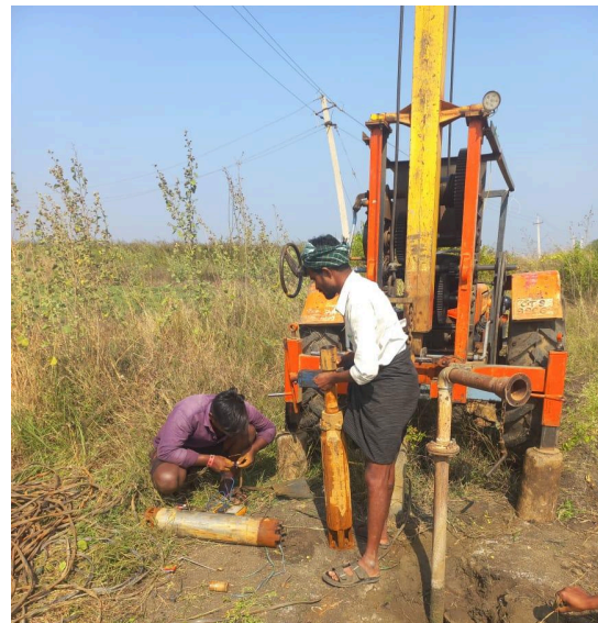
Action 10: Pipeline and motor being repaired at Chikkapanahalli
