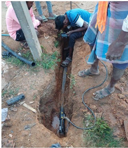
Action 13: Drinking Water Pipeline repaired in M Hosahalli
