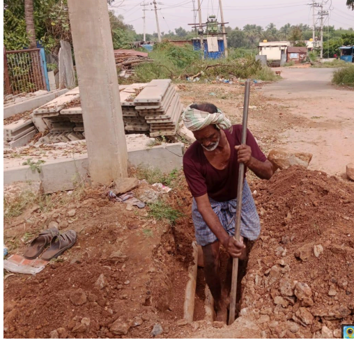
Action 9 : Repairing of drinking water pipeline at Ramajogihalli
